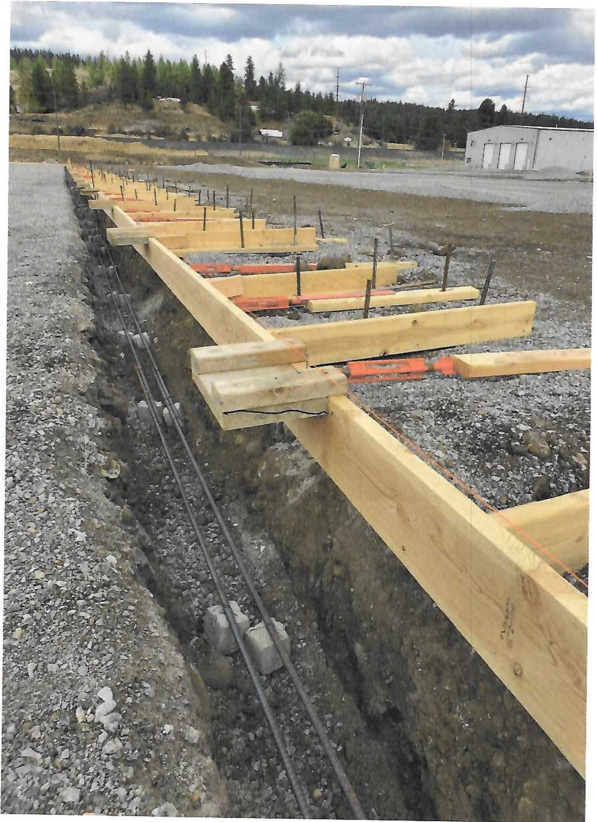
Figure 3 Forming Mullion Notches
