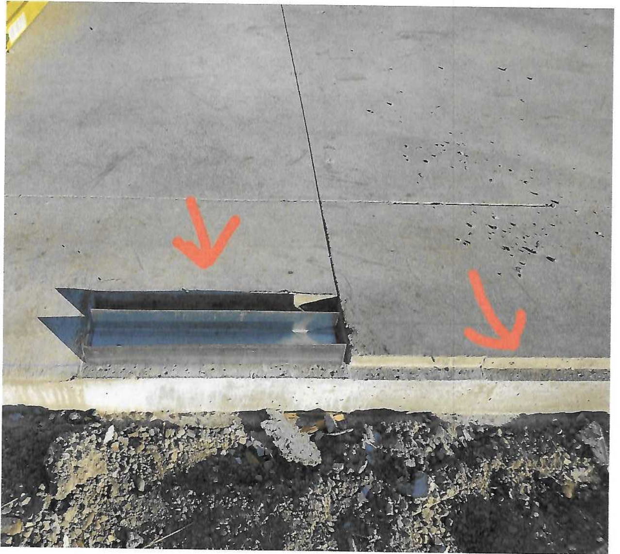
Figure 5 Mullion notch and PBR 1.5" channel
