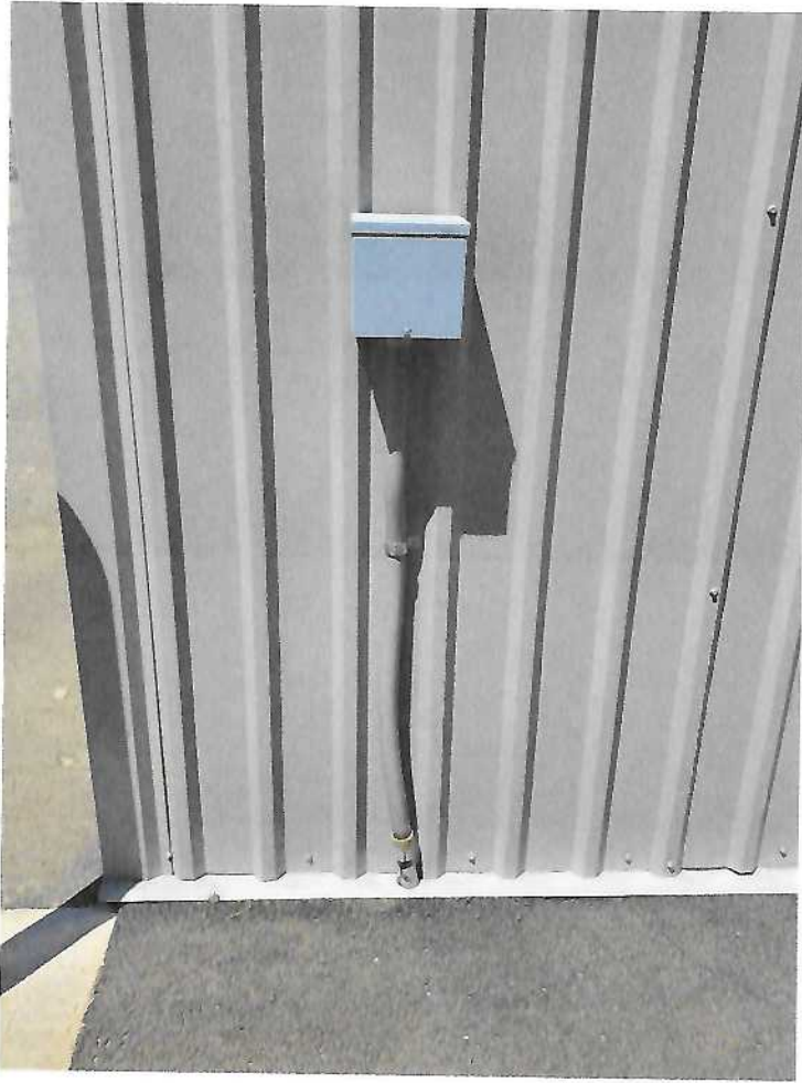
Figure 2 Drip edge with no overpour
