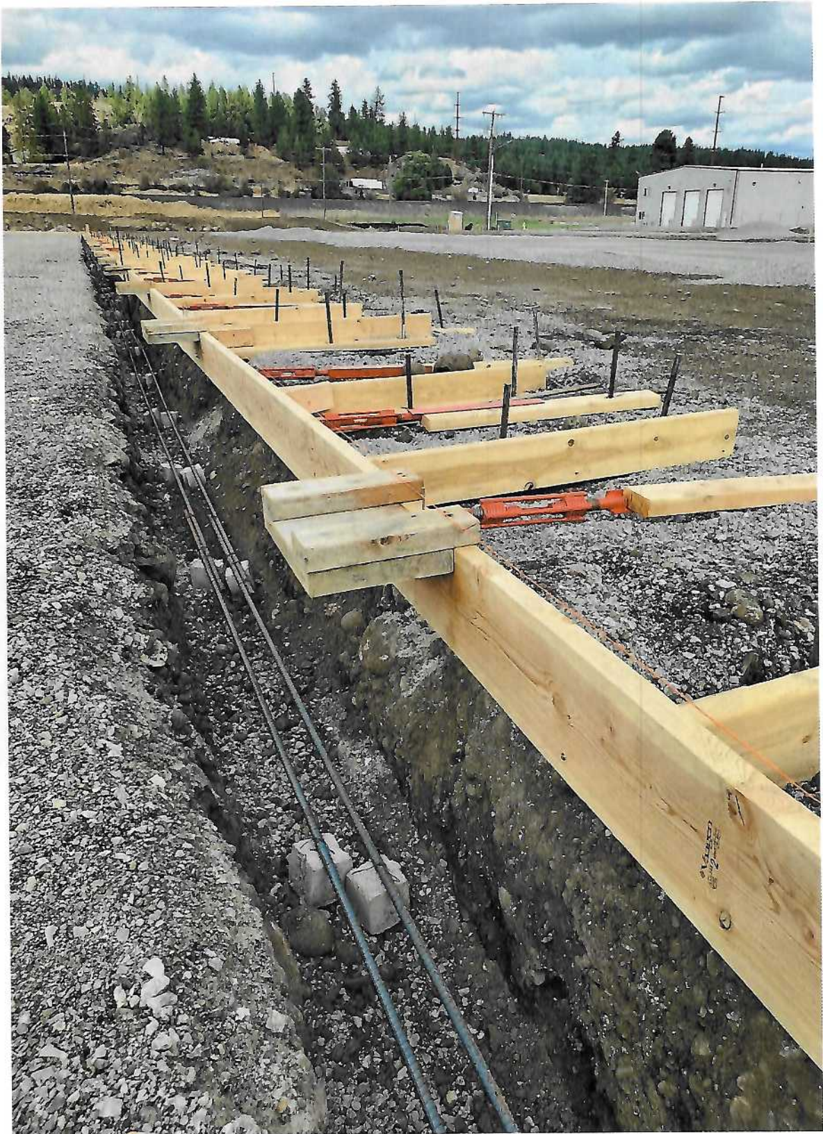
Figure 3 Forming Mullion Notches
