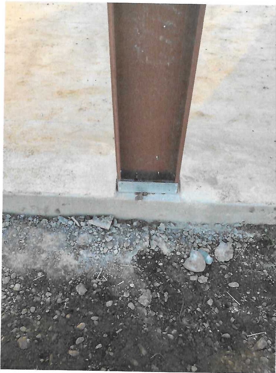
Figure 6 Mullion notch with Channel and Column
